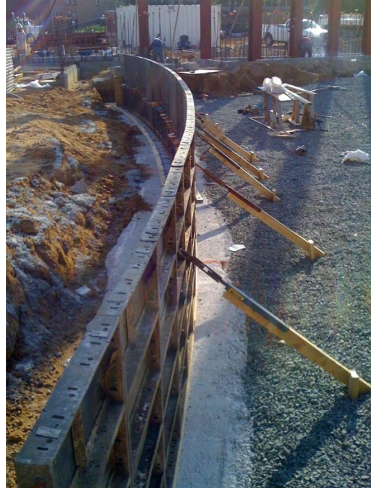
Figure 4: Auditorium Form Work @ Stage Wall
