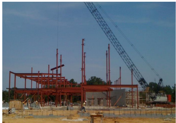
Figure 3: Steel Erection Section F
